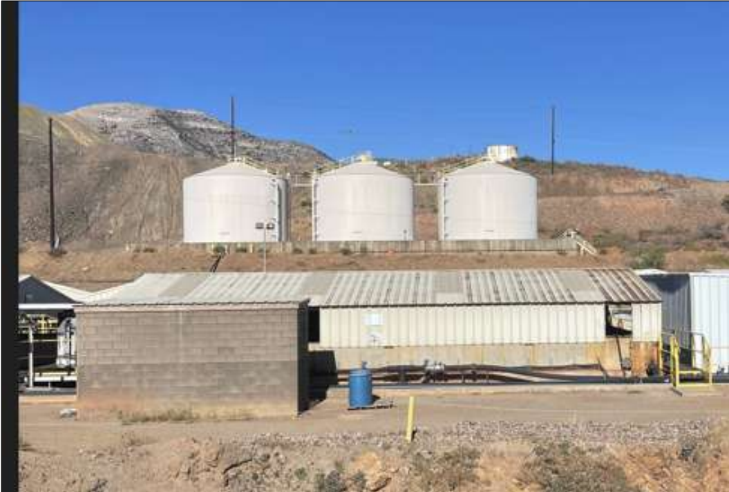
Figure 17-13: JCM Sulfuric Acid Tanks
