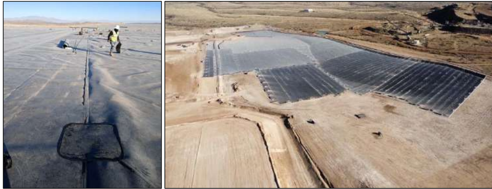
Figure 17-4: Liner Installation on Pad 5
